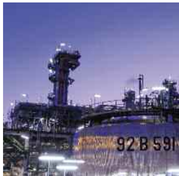
Total's combined cycle CHP station in Gonfreville, France.
